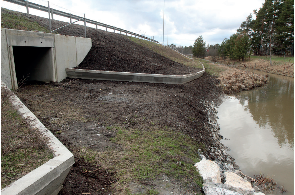
Fig. 61.4 Amphibian tunnel at Merkja (Nordre Øyeren Nature Reserve) illustrating extensive foraging areas out of reach for amphibians. The prevention of communication between researchers from the EIA and mitigation stages of the road resulted in unnecessary mistakes. Also, there was a lack of a buffer zone between the terrestrial and aquatic habitats. The fence and tunnel should have been placed higher up on the slope. Mitigation failed to include replacement habitats. Photograph by Leif Yngve Gjerde.
